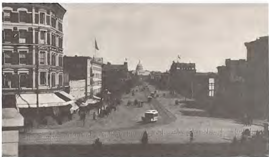
View from Treasury Building to Capitol showing Cosmos Club quarters, 1879–1882, on third floor of Corcoran Building at northeast corner of Pennsylvania Avenue and 15th Street, NW.
