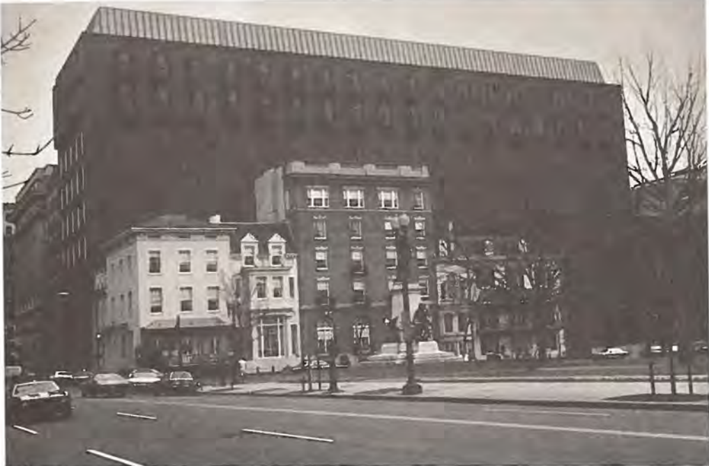
Former Cosmos Club quarters today (1978) at H Street and Madison Place, with new Court of Claims building in background.
